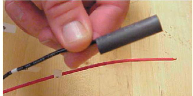
7. Use a heat source to seal the heat shrink. Insure the wire insulation has no signs of overheating or mechanical damage.
