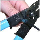
3. Be sure all wires are cut to the same length and fully inserted into the crimp connector. If crimping is performed with only a few wires exposed to the device, it will lead to a loose or weak connection due to a reduction in current carrying capacity. Just like a weak link in a chain will make the whole chain weak, a poor splice connection will weaken the entire length of wire.
